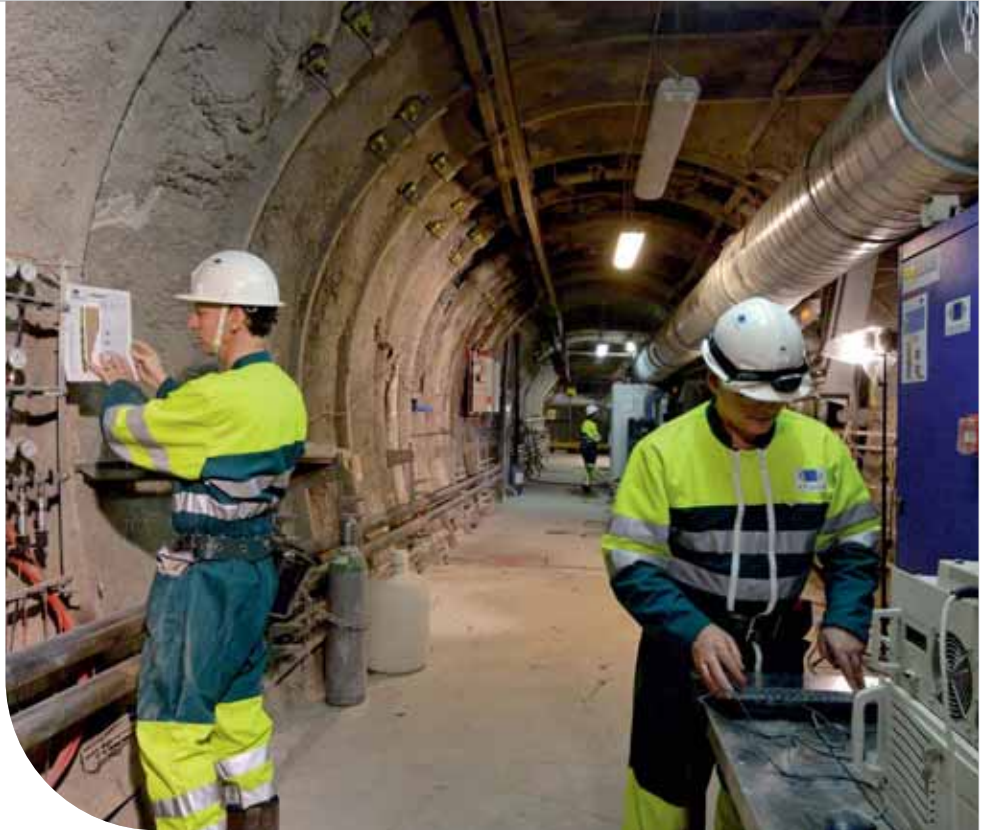
▲ Experimental tunnels at Andra's underground research laboratory in Meuse / Haute-Marne, east of Paris.
