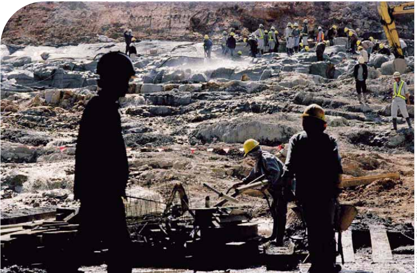
▼ Nam Theun Dam construction site, where 2,500 people work, of which 80% Laotians.
